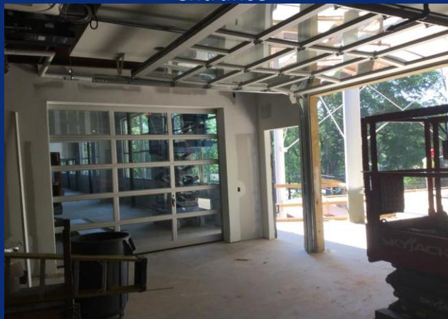
Overhead door installed in STEM lab
