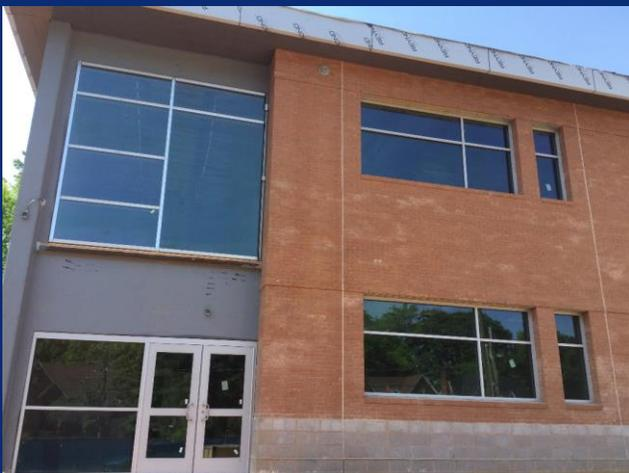
Store front doors and windows installed at East stair
