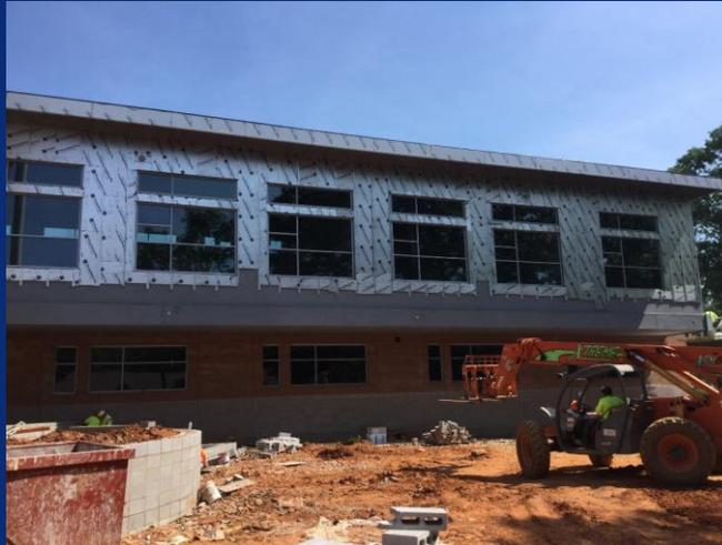
Metal panel insulation in progress on elevation 1
