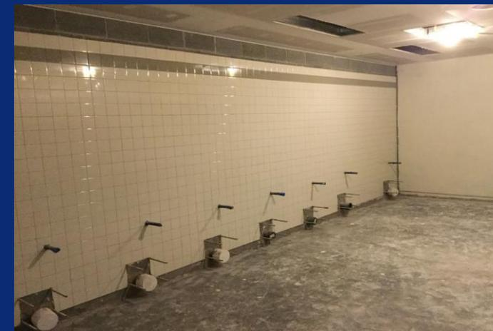
Ceramic tile in progress in main level restrooms
