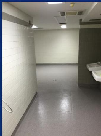
Epoxy flooring complete in lower level restrooms
