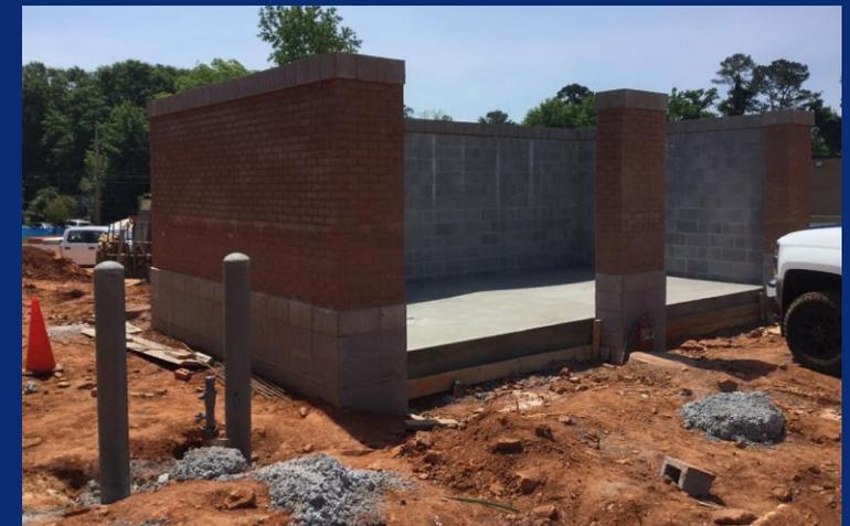
Dumpster pad brick complete and slab poured
